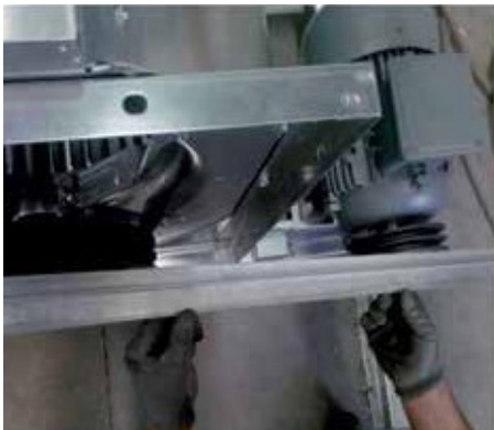
Image 6. Alignment Check of Pulleys-1
