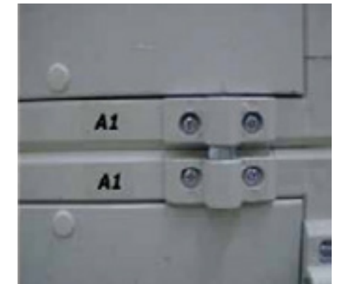
Picture 3. Cell joining
