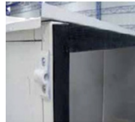
Picture 1. Sealing gasket between cells
